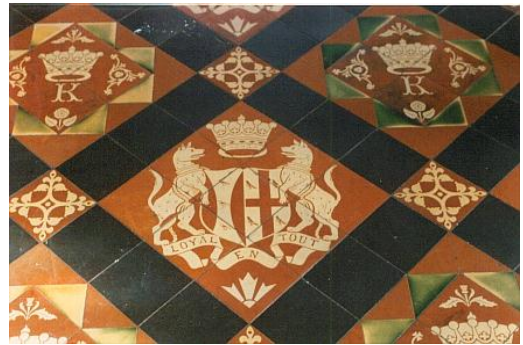
The Kenmare arms set in encaustic tiles, Chapel, Killarney Cathedral
