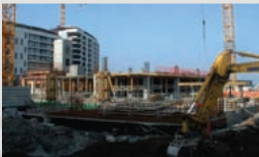
Building Progress at March 2009
